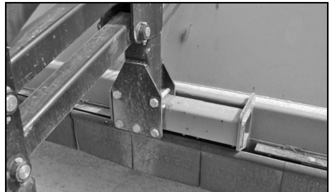
Figure 46. Strut Uprights Installed
